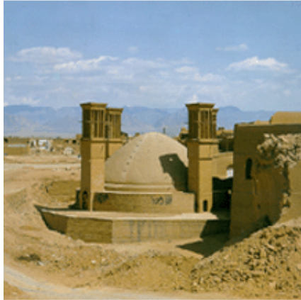
Figure 2-5. A traditional Iranian building. The desert buildings are equipped with air traps, arched roofed, water reservoirs with arched domes and ice stores for the preservation office.
