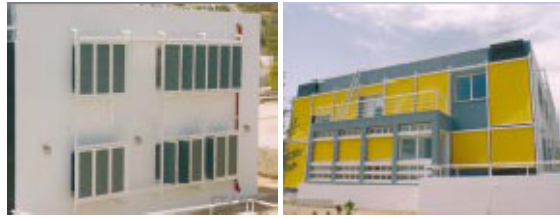
Figure 1-10. Sun protection systems on the south and east facades
