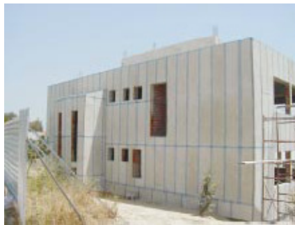
Figure 1-8. External insulation on the north face of the building
