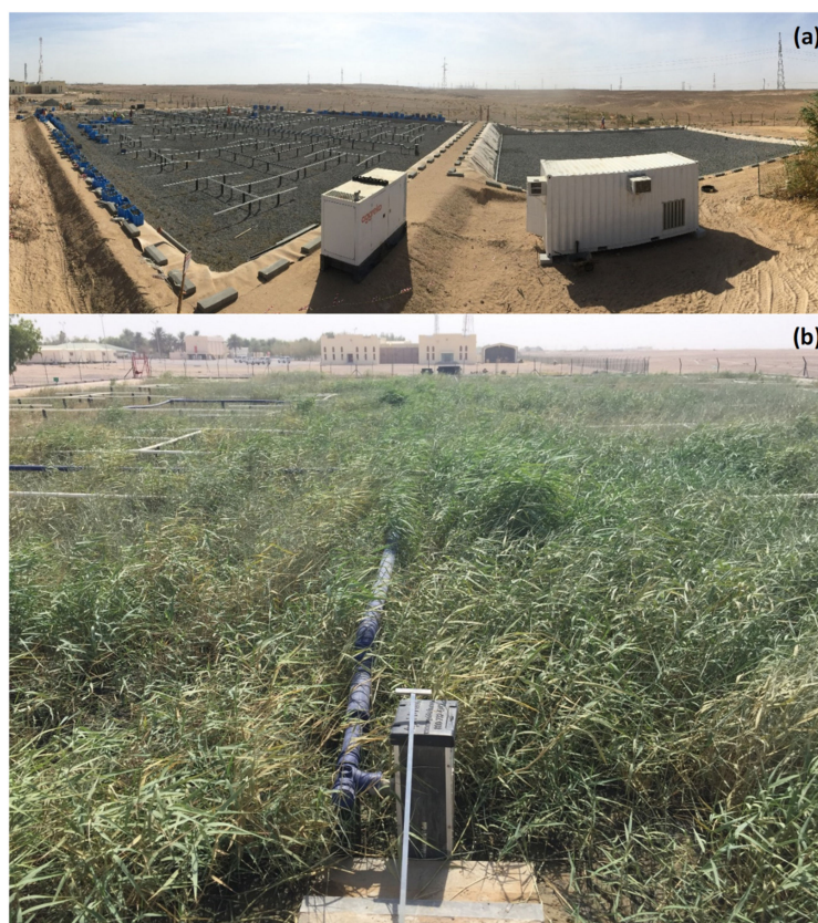
Figure 5. (a) Aerial view of the two-stage Constructed Wetland in Oman during plant establishment, comprising a first stage vertical flow CW and a second stage aerated horizontal flow CW, followed by UV disinfection, and (b) the first stage VFCW one month after initial planting ([57]; Courtesy of Bauer Nimr LLC).
