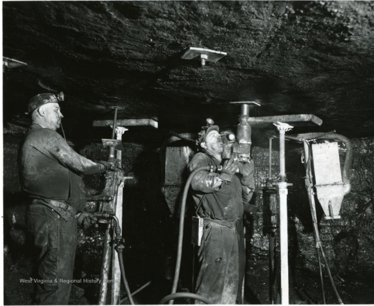
Σχήμα 13. Bolting (Consolidation Coal Company. Bishop Mine, 2020).
