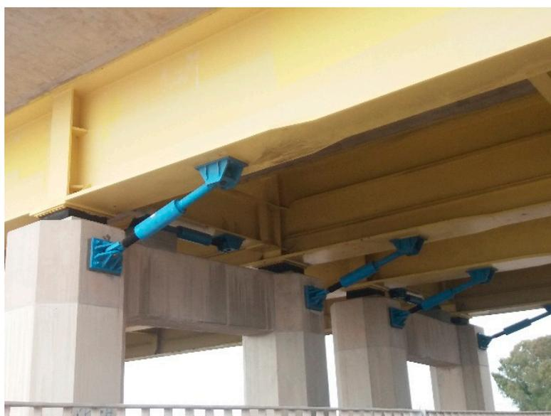
**Figure 1.** Supplemental viscous dampers installed in conjunction with elastomeric bearings in Rion-Antirion bridge, Greece.
