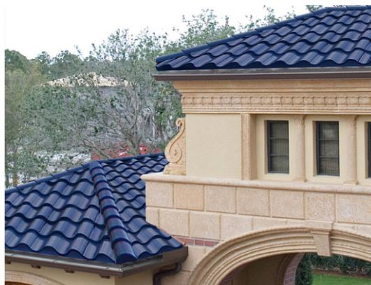
Figure 1.11: Sole Power-Tile integrated on a building roof.
