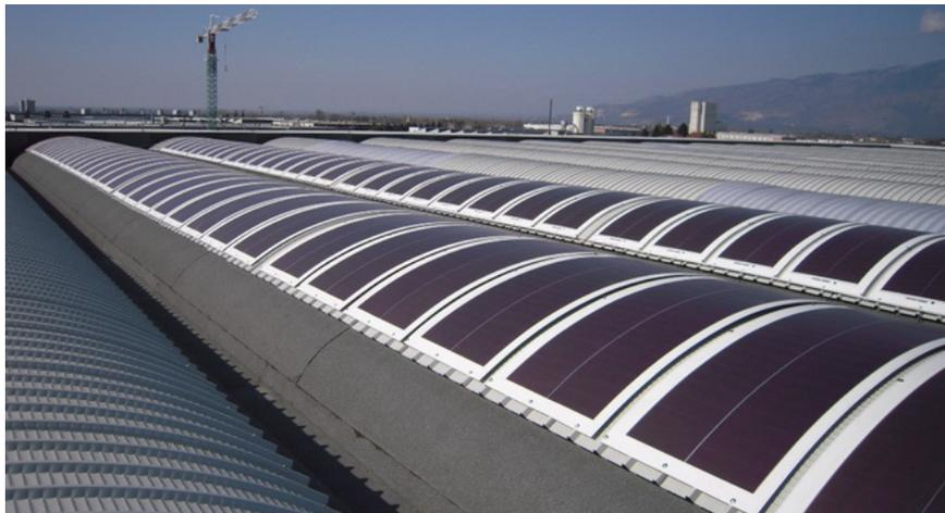
Figure 1.13: PV flexible modules installed on curved roof
