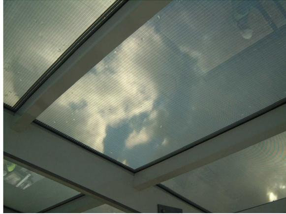
Figure 1.9: BIPV module based on thin-film technology.
