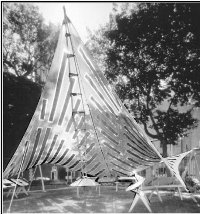
**Fig. 5.6.** Thin film module (are flexible and are easily integrated into curved surfaces) (Lechner, 2001)
