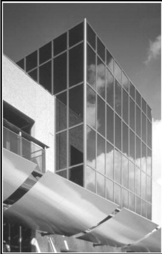
**Fig.5.2.** The APS building in Fairfield, California, USA. Thin – film PV technology integrated into curtain wall system. Curtesy Kiss and Cathcart architects. (Lechner, 2001)
