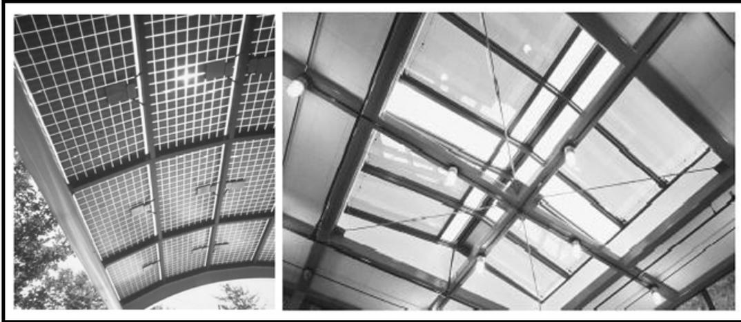
**Fig.5.4.** Opaque PV cells mounted on clear glass. The space between the cells determines the degree of shading. Aquatic Center at Georgia Institute of Technology, (left). Semitransparent PV glazing as skylight glazing in APS Factory in California, Courtesy Kiss and Cathcart, architects (right). (Lechner, 2001)
