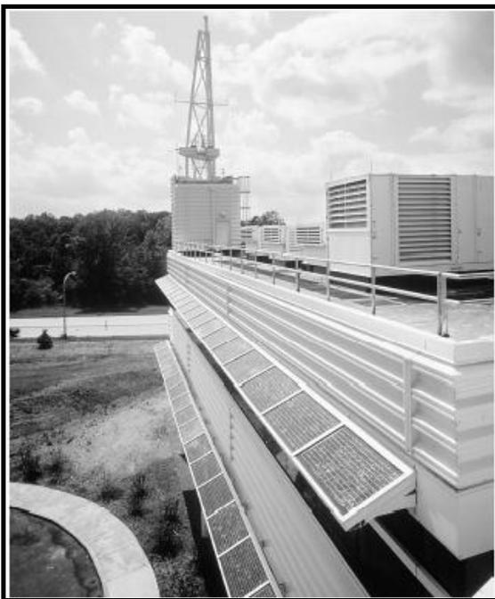
**Fig.5.3.** Tilt PV shading Devices in Center for Environmental Sciences and Technology Management building (CESTM) in New York, Courtesy Kawneer Company Architects. (Lechner, 2001)
